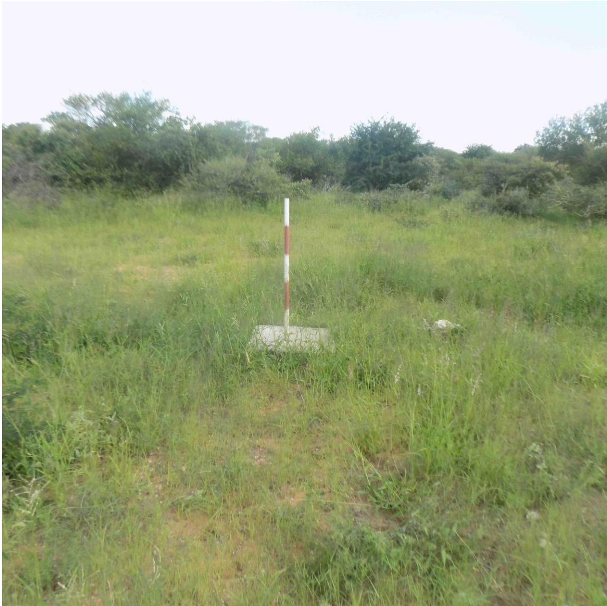
Figure 5.5: Completed and rehabilitated drill hole
