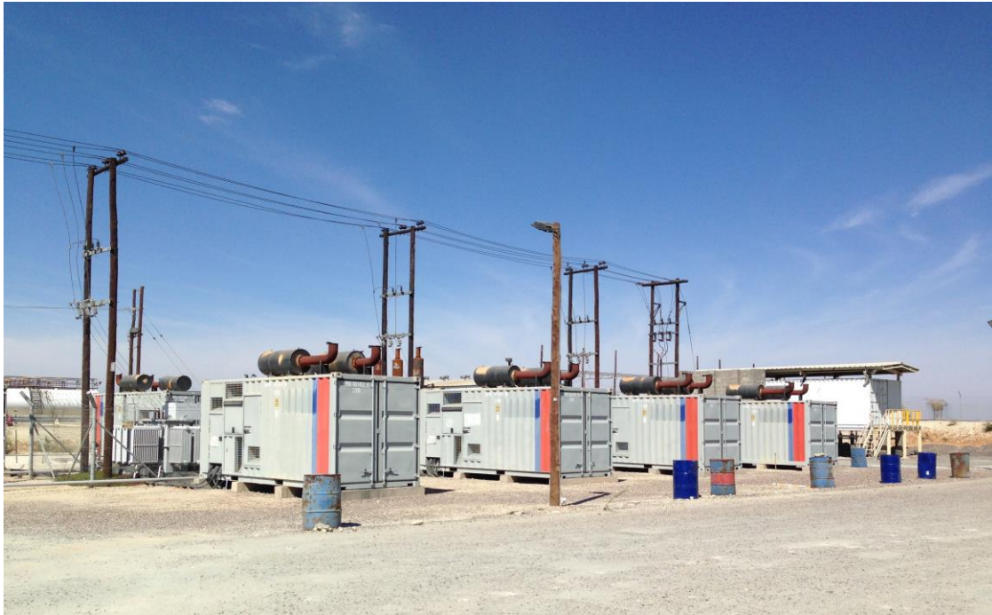
Figure 2.16: Example of on-site diesel power station (Source: APR Energy website)
