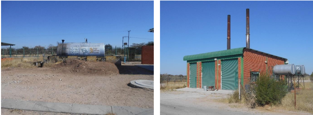
Figure 5.39: Used oil storage container and incinerators at the Ghanzi landfill
